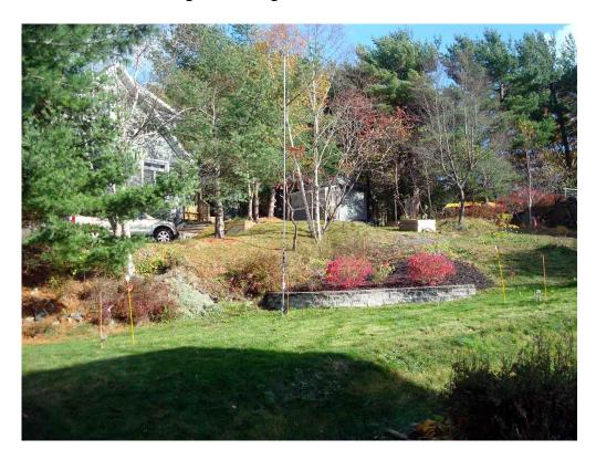
The yellow stakes are fiberglass snow markers which are used to hold up the ends at the correct level. They are bent slightly to preload the tension on the guys and keep everything snug with a bit of spring. We just went through a storm with 90 KPH winds with no problems.
